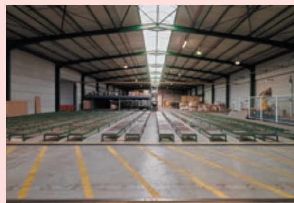
One of Bauwens production halls before the refurbishment project had started.
