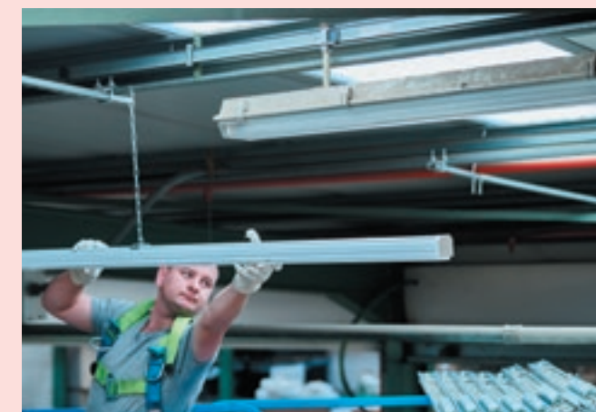
Light refurbishment without production downtime.
